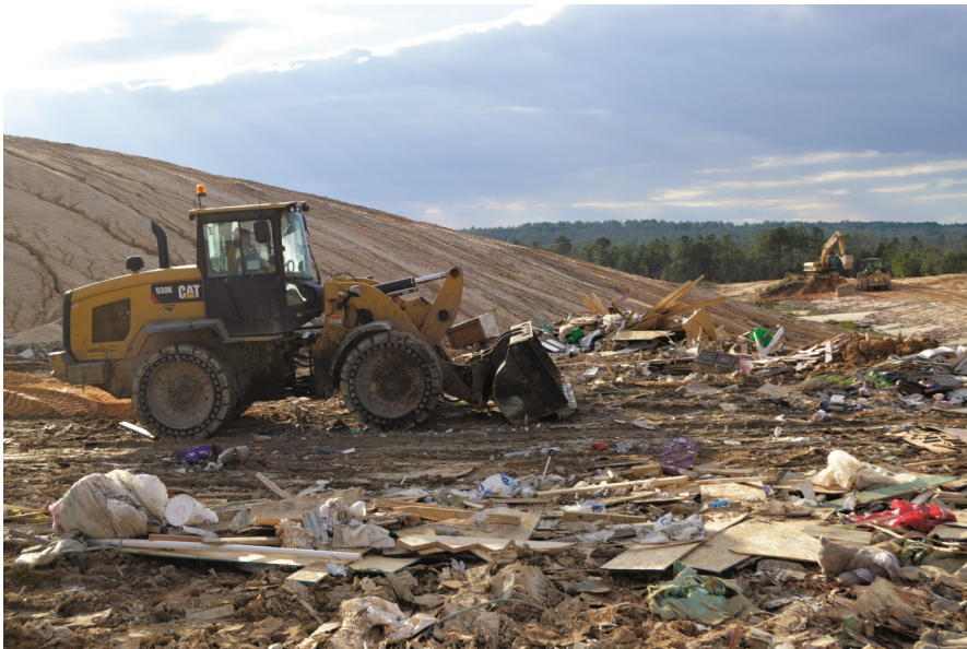
Employees with Harnett County Solid Waste work at the Anderson Creek Landfill where they the department is constructing a new cell that will last the county five more years.
